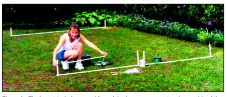
Figure 6—The layout technique used for quick wire measurement and assembly of the loop and its associated hang-up harness. Note the use of PVC pipe stakes, carefully positioned and squared, for forming the structure. Both the 17 and 10 meter elements can be put into place during this operation.
